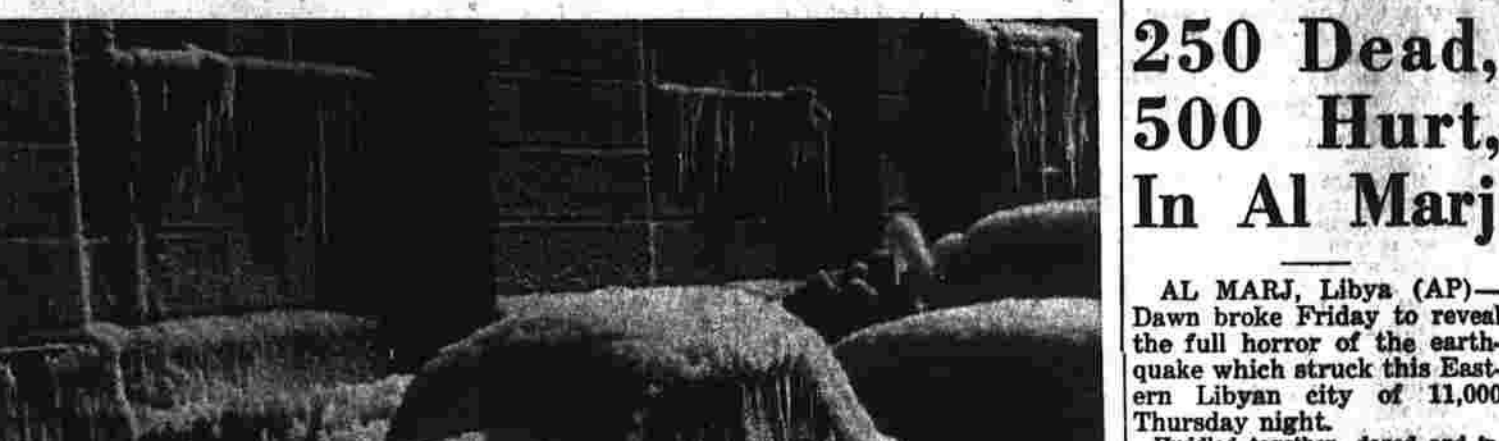
In the aftermath of yesterday's fire cars along Ann St. were thickly coated with ice and frozen to the ground.
